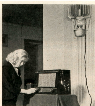
Kerosene Radio Made in Moscow for use in rural areas, this all-wave radio is reportedly powered by the kerosene lamp hanging above it. A group of thermocouples is heated internally to 570 degrees by the flame. Fins cool the outside to about 90 degrees. The temperature differential generates enough current to operate the low-drain receiver. Regular listeners may want fur-lined union suits, though: It works best in a room with open windows.
